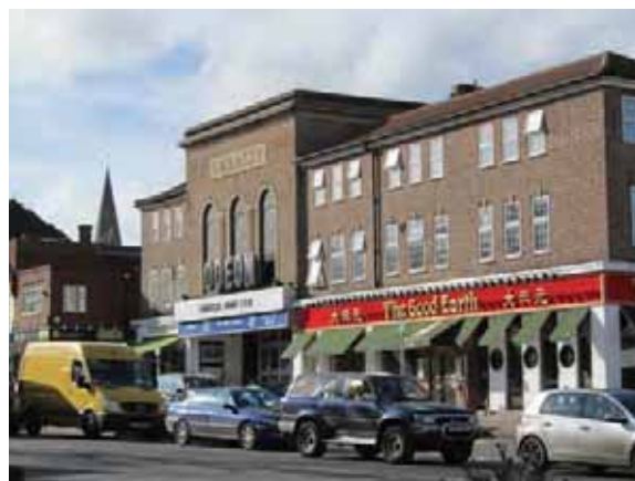
Mixed use development to High Street, Esher
