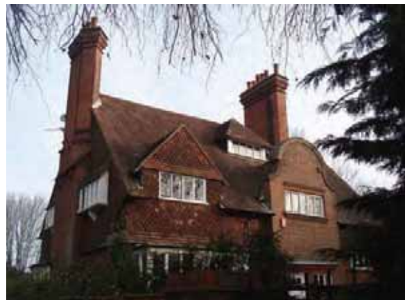
High end Domestic Revival, Oatlands Drive
