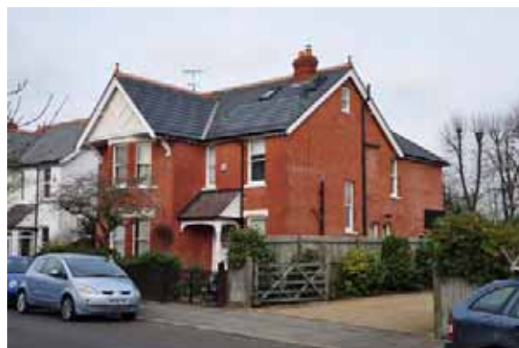
Solar panels on traditional roofslope
